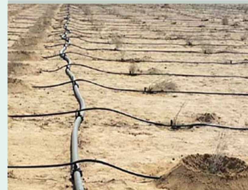
• A side of the soil reclamation after cleaning the oil pits in WJO
